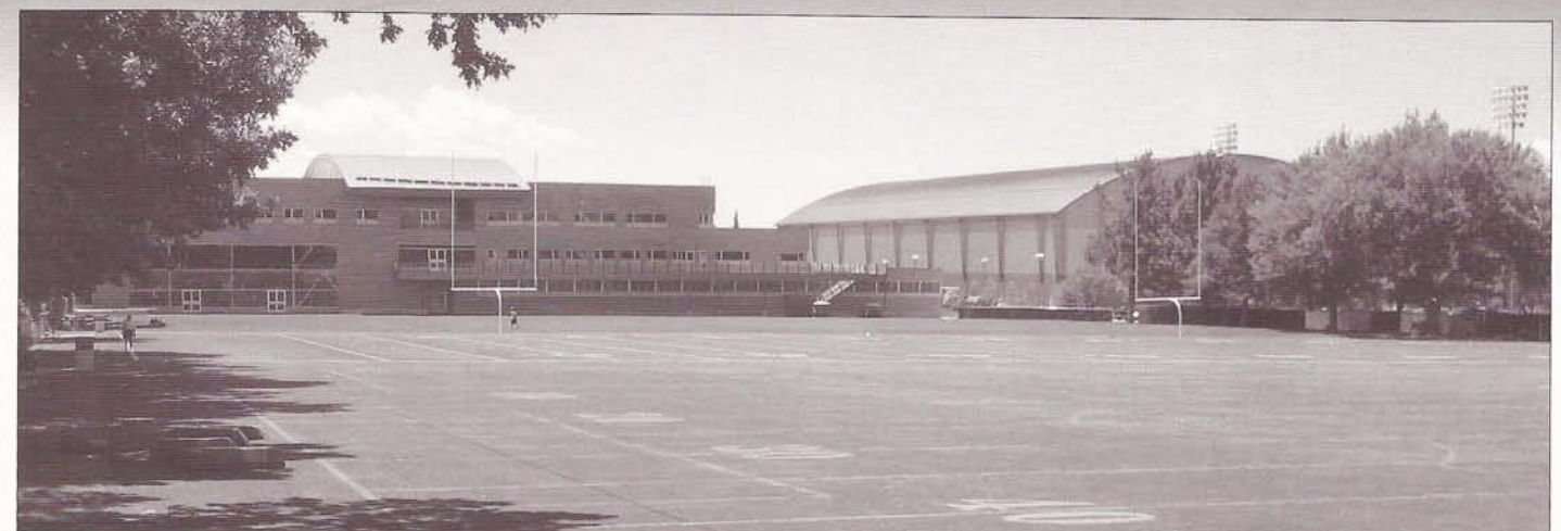
View of new Student Athlete Building and Indoor Practice Facility from football practice field
