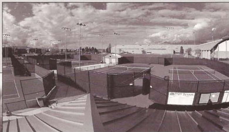
Adjacent to BYU's recently remodeled outdoor tennis complex is BYU's South Field—home of BYU's men's and women's soccer teams—and the Smith Fieldhouse. The Smith Fieldhouse contains facilities for nearly every sport, including a one-fifth mile rubberized track that surrounds three basketball courts and an artificial turf practice area.
