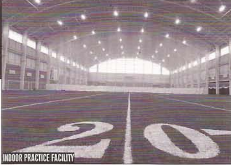
INDOOR PRACTICE FACILITY
